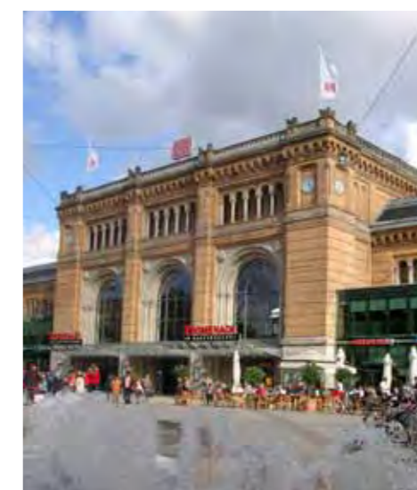
ECE also has expertise in the refurbishment of transport properties as demonstrated, for example, at Hanover Central Station.
