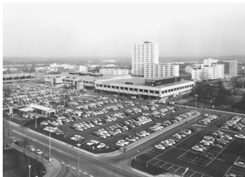
ECE's first own shopping center, Franken-Center in Nuremberg, opened on October 23, 1969.
