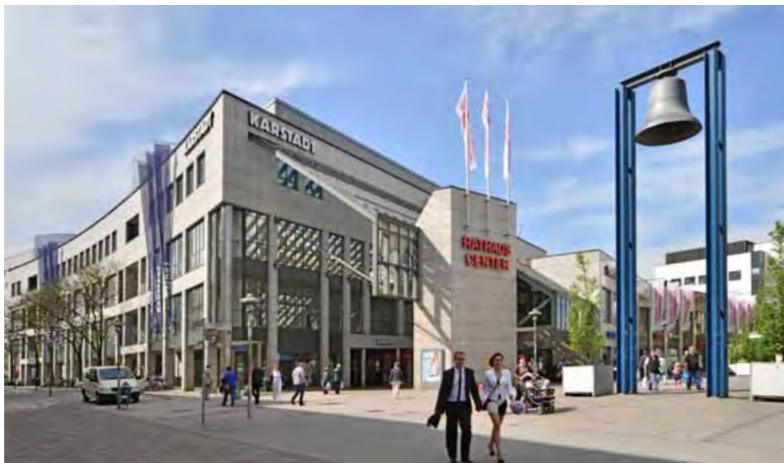
Rathaus-Center in Dessau was one of the first shopping centers that ECE opened in the new federal states.
